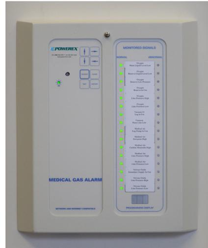
Master alarm conversion shown above is 16 signals – part # PX-DU716
